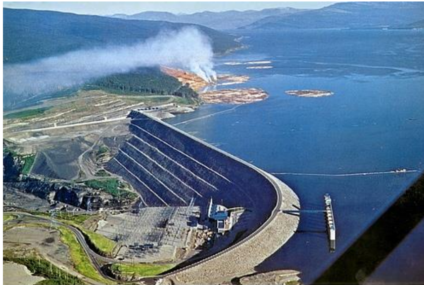
Bennett Dam, B. C.
